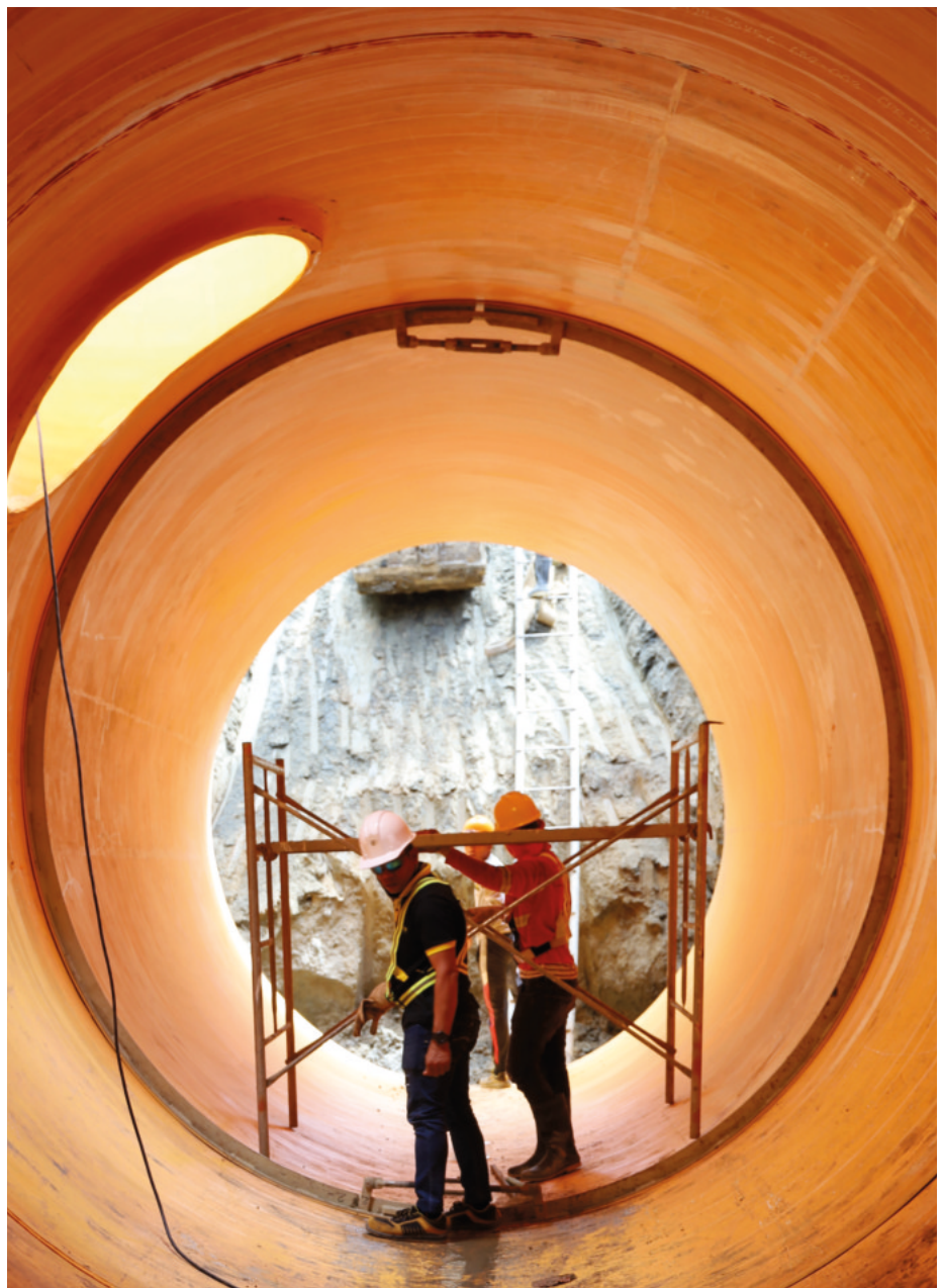
Inside the pipe in the trench
