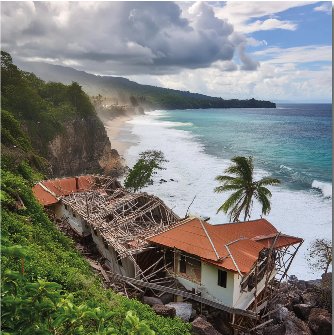
AI-generated symbolic picture of a damaged house caused by an earthquake in the Philippines
