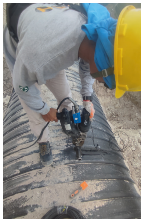
Siphon 4 Inlet - Repair works
