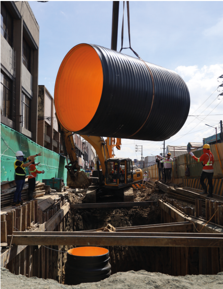
The DN/ID3500mm Krah pipe „flying“ over the construction site
