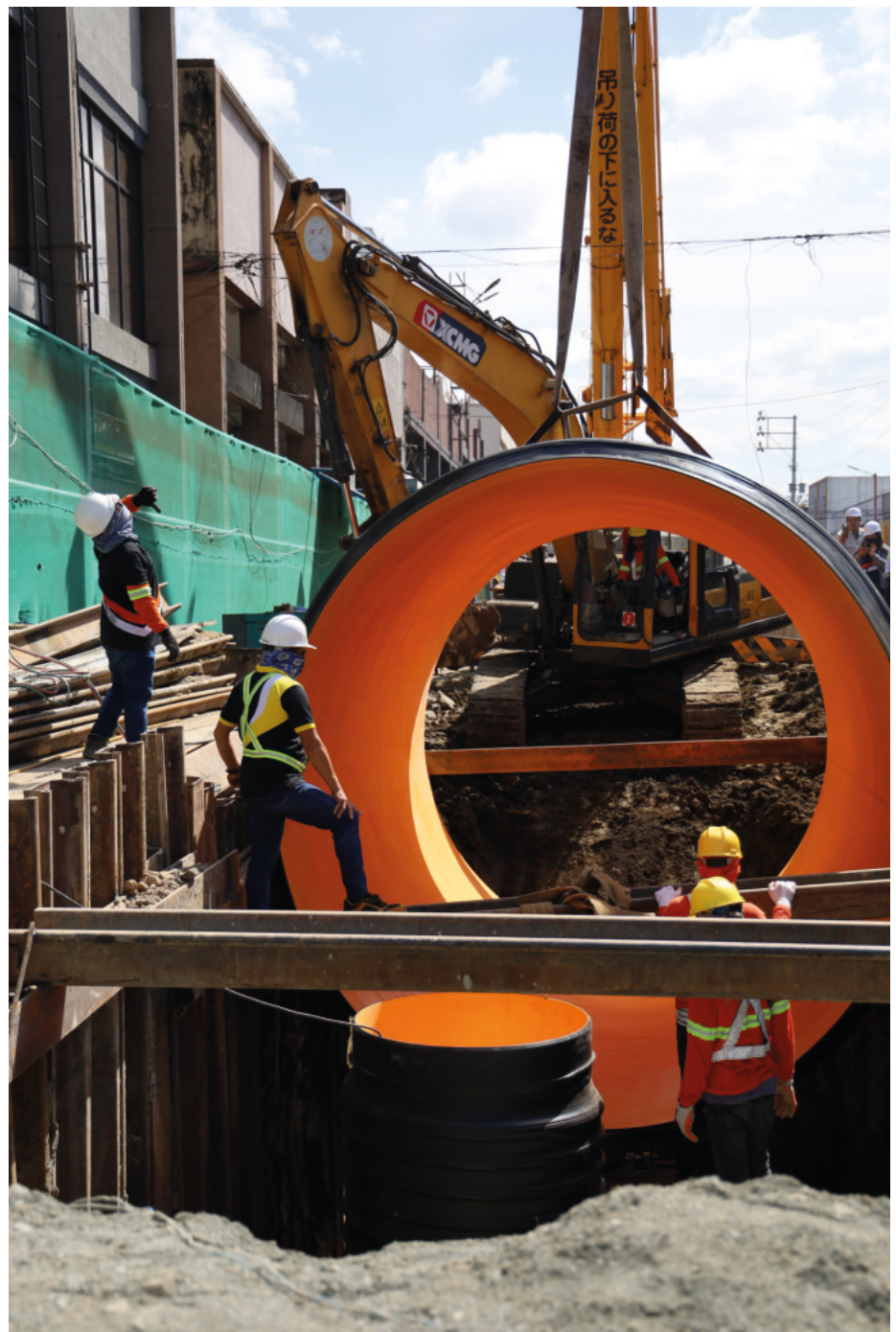
Lowering the pipe into the trench
