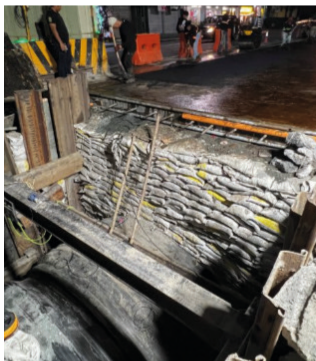
Backfilling and compaction
