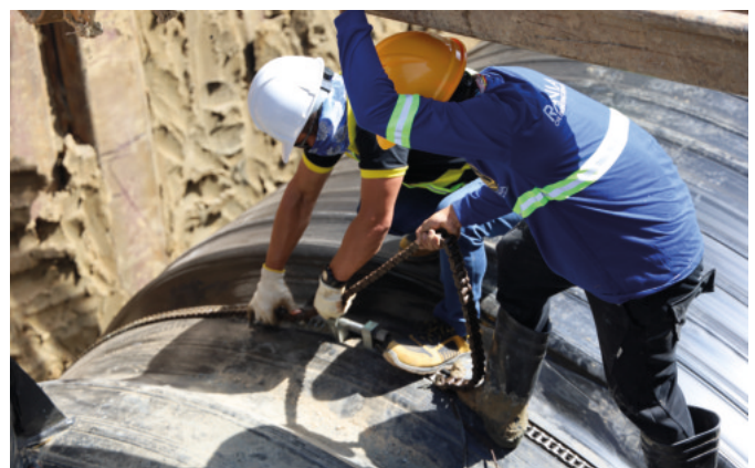
Tightening the chain around the pipe for electro-fusion
